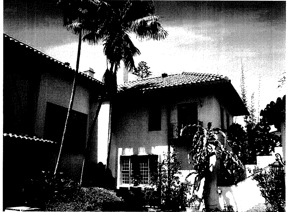
Existing Property - View from rear courtyard of the northeast elevation of the Main House. Visible on the right of the photo is the existing exterior stair connecting the Main House with the Caretakers' Cottage.
